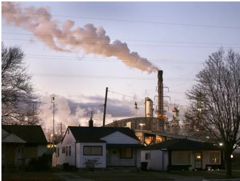
The Marathon Petroleum refinery operates in the background of a residential neighborhood in southwest Detroit. (Photo: Romain Blanquart, Romain Blanquart/Detroit Free Pr)
